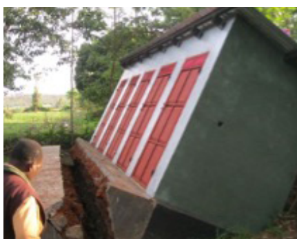
Fig. 2: Collapsed School Toilet Building after Heavy Rains, Tanzania (Photo: source unknown)
