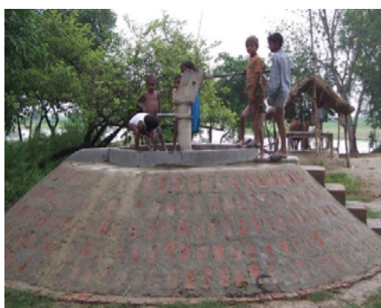
Fig. 3: Flood-proofed handpump in Bahraich, India: the apron is elevated one meter high and the slope of the base gradual enough to prevent damage during flash floods (Photo: District Administration, Uttar Pradesh, India)
