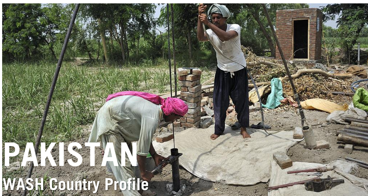
After the devastating floods in 2011, WHH introduced manual drilling in the flood affected areas in Punjab. ©Kopp
