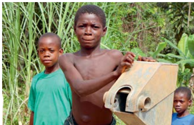
A broken hand pump in Solo Town, Liberia. An estimated 30 percent of installed hand pumps in Africa are non-functional and another 40 percent are only partially working, on average, after three to five years of installation.
